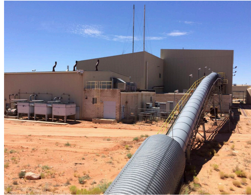
Shootaring Canyon Mill in Utah (Quelle: Anfield Energy)
